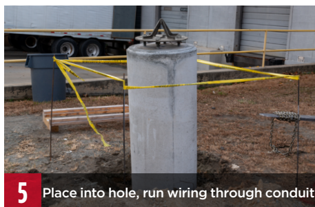
2 Attach lifting bracket to pole base.
