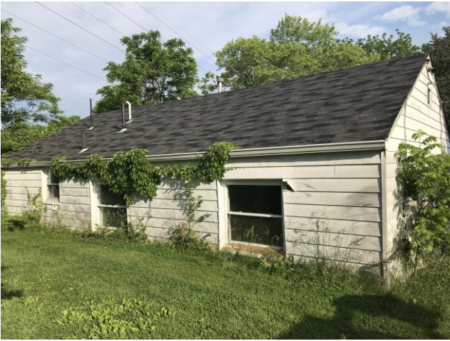
Location of Samples 227-1-1 (shingles/felt), 227-3-1 (fiberboard under siding) and 227-4-1 (window caulk)
