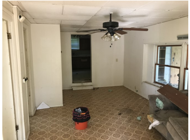
Location of Samples 227-5-1 (ceiling tile), 227-6-1 (linoleum) and 227-12-1 (fiberboard ceiling panel)
