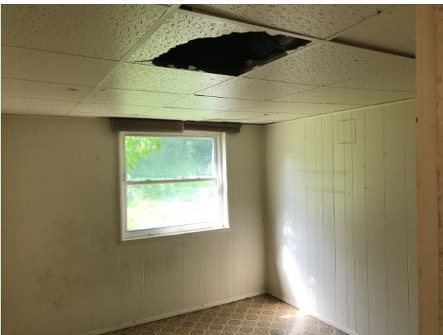
Location of Samples 227-5-2 (ceiling tile), 227-6-2 (linoleum) and 227-12-2 (fiberboard ceiling panel)
