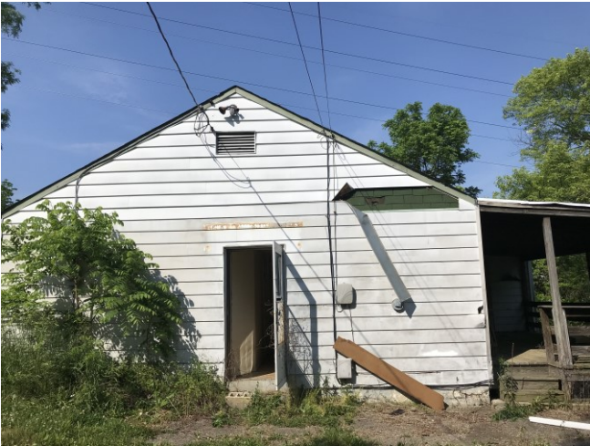
Location of Samples 227-15-1/2 (shingles under siding) and 227-16-1/2 (fiberboard under shingles)
